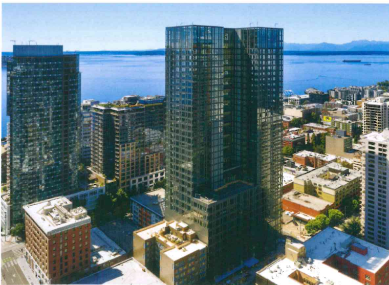
Third and Lenora is a 36-story office and apartment tower in Seattle, Washington State. The complex was designed by Perkins & Will of Seattle. Guardian SunGuard SuperNeutral 68 coated glass was used to help maintain the building’s climate control. This mixed-use project was honoured with a Commercial Project Award by Guardian Glass in 2021. Photograph produced by Clarity Northwest Photography and provided courtesy of Guardian Glass, August 17, 2020.
