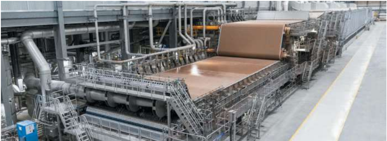
The new machine (called the “Marguerite K”) uses, on average, only 140 gallons of fresh water per ton, most of which goes to critical applications like boiler feed and system cooling.
