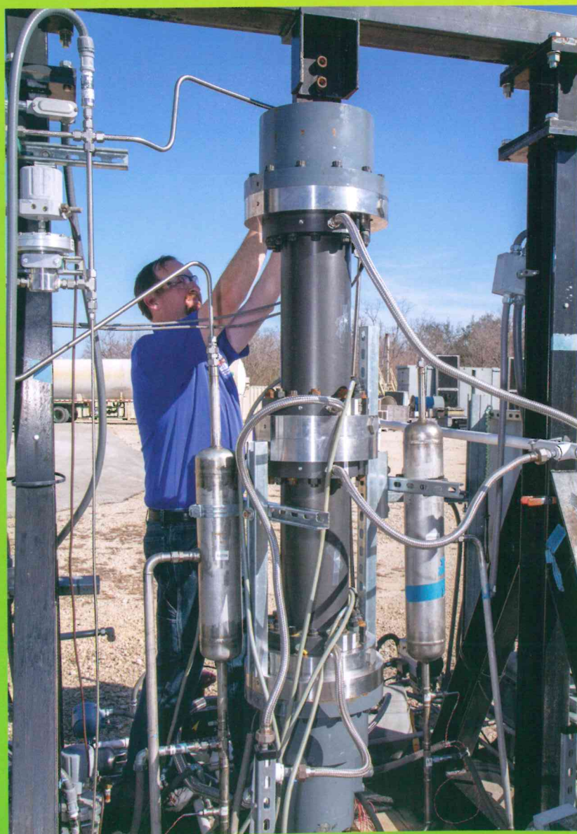
Senior Research Engineer Nathan Poerner performs maintenance on the hermetically sealed LMRC that SwRI designed for hydrogen compression.
