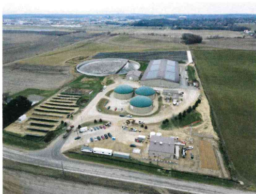
2. EnTech Solutions owns and operates a biodigester facility in Middleton, Wisconsin. A majority of the facility's power comes from an onsite solar-plus-battery microgrid. Courtesy: EnTech Solutions
