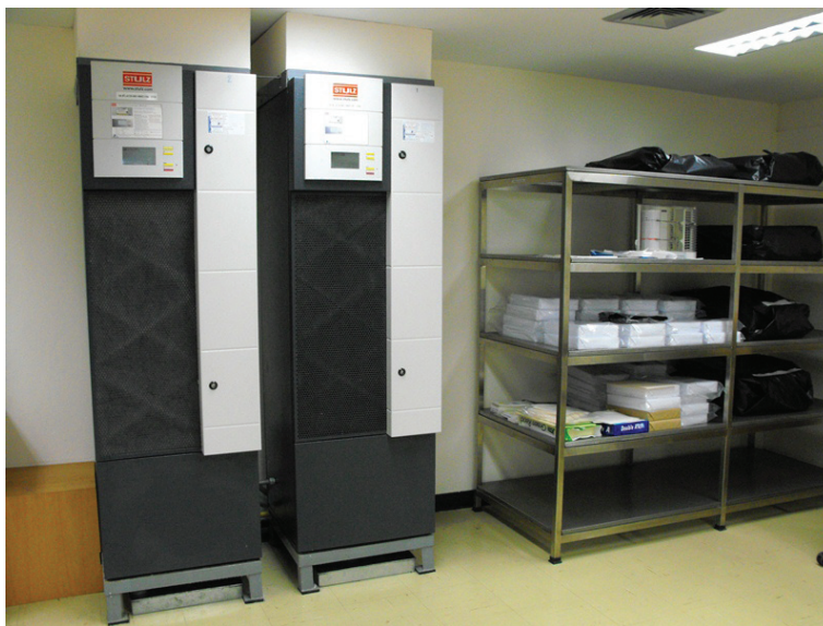
Figure 11 Pulp and paper subdivision of the Physics and Engineering division of Department of Science Services' Optical laboratory. The temperature is controlled at 23 \pm 1^{\circ}\text{C} and the humidity is controlled at 50 \pm 2 percent for 24 hours per day.
