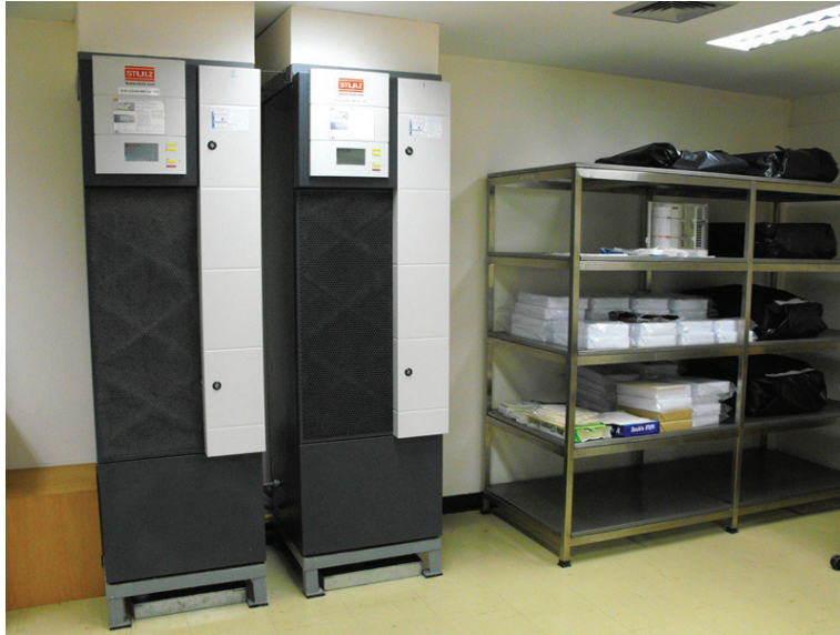
Figure 11 Pulp and paper subdivision of the Physics and Engineering division of Department of Science Services' Optical laboratory. The temperature is controlled at 23 \pm 1^{\circ}\text{C} and the humidity is controlled at 50 \pm 2 percent for 24 hours per day.
