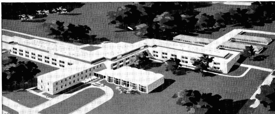
Research and development building at Cyanamid's Agricultural Center
