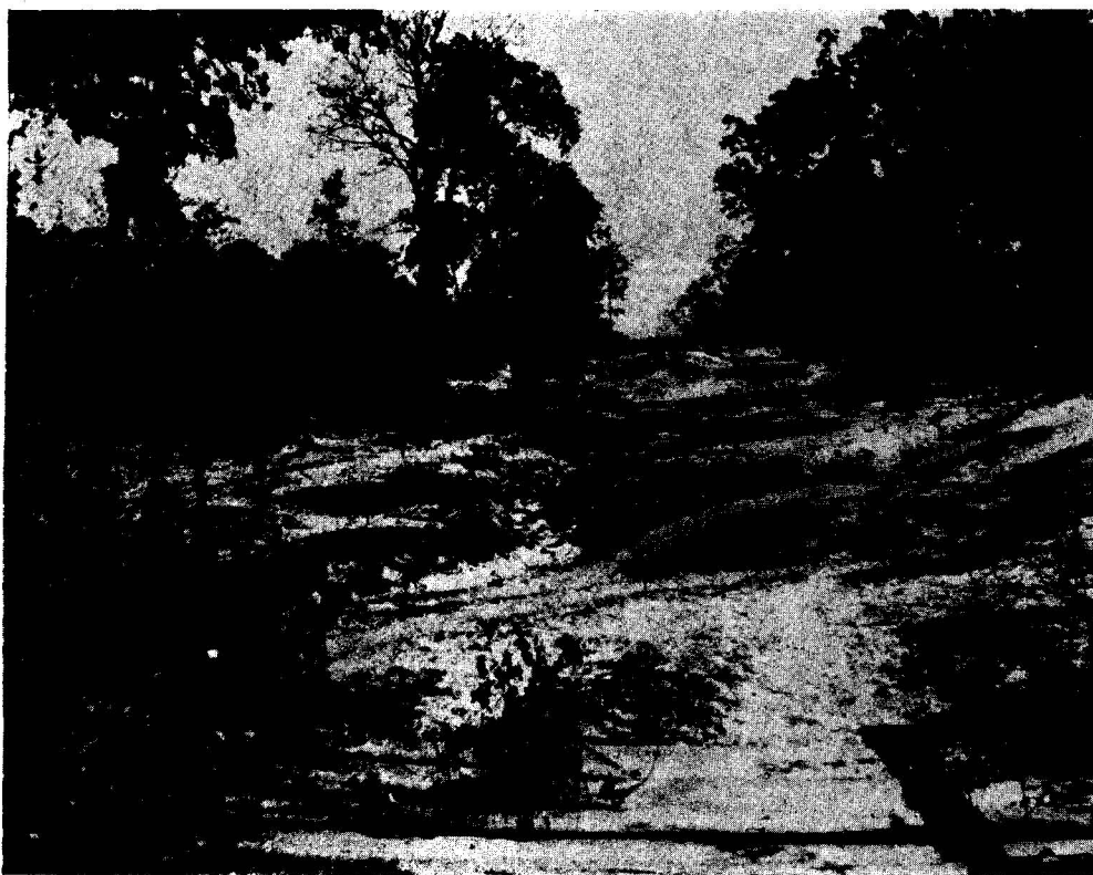
Fig. 6. From the bridge in the foreground, looking up the slope of the road. Much of the fine sandy white lixivium soil has been eroded from this road, exposing as darker patches the iron concretions washed clean by the beating rains. The shallow gullies are eroded to the massive laterite, which was sampled (871-L) in the middle distance. (cf. preceding Fig. 5). Wang township (อ. แวง), Roi Et Province (จังหวัด ร้อยเอ็ด), Northeastern Thailand. March 1940. RLP Foto 1232—6.
