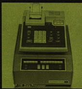
AUTOMATE. Expand Spectronic Spectropho-tometers to automated sys-tems with data printer, sampler for unattended operations, diluter-pipetter for sample, creagent dis-pensing. Lets you identify samples, consume less reagents, all automatically.
