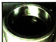
Filled boiling vessel ready for startup
