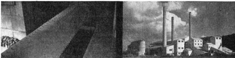
The new cement mill
