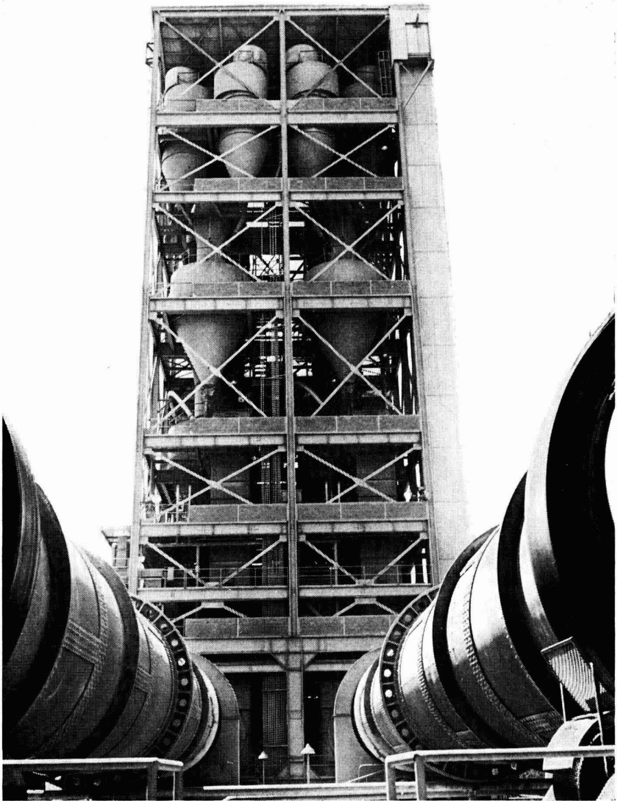
Fig. 1.—The Two Kilns and Preheaters.
