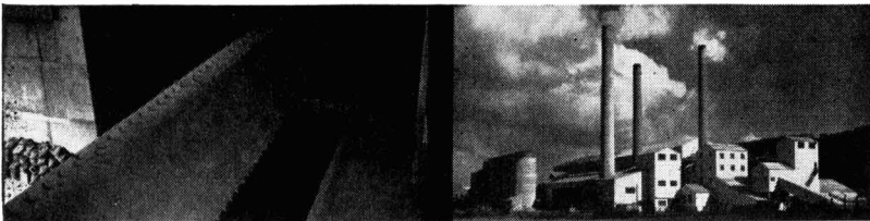
The new cement mill
