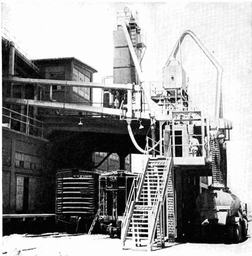
Fig. 4.—Loading Loose Cement.
