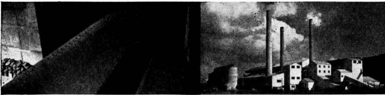
The new cement mill
