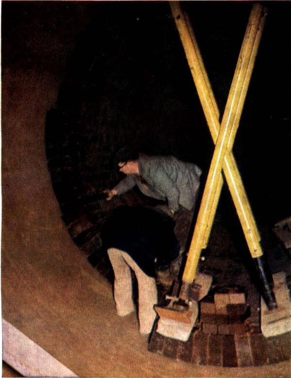
Kiln lining in progress with Magnesite/Chrome bricks
