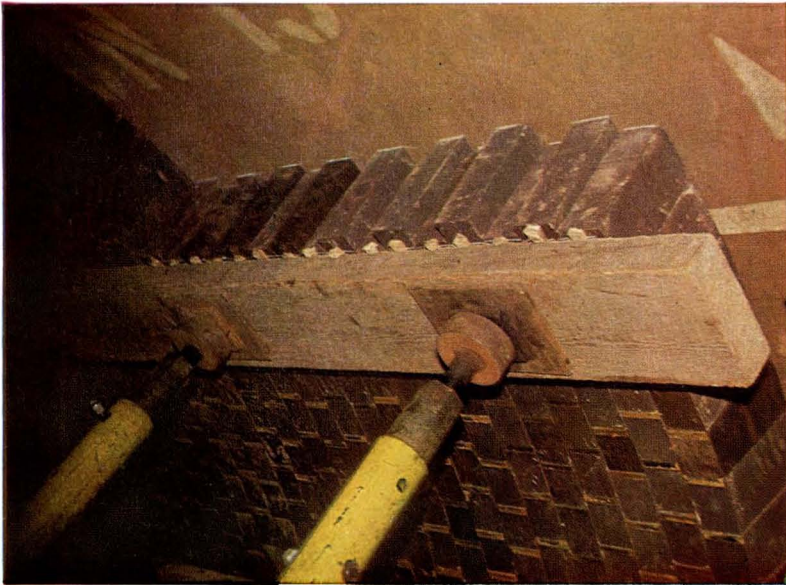
Illustration shows details of Jack assembly
