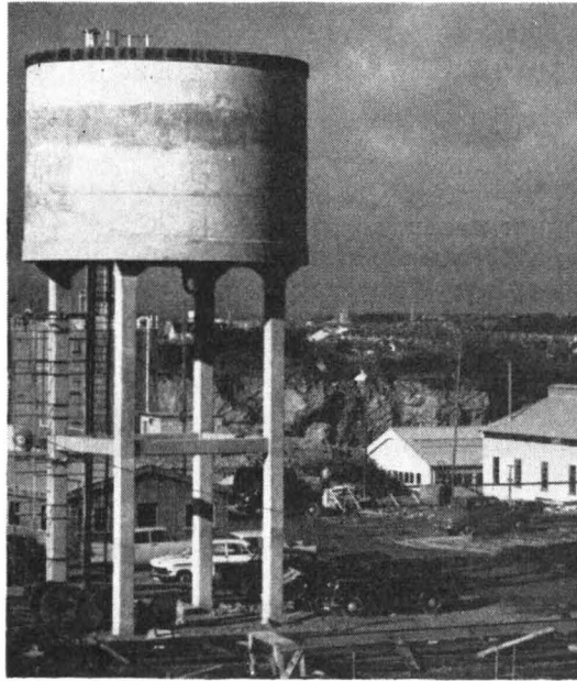
Fig. 14.—Water Tower. (End of Kiln House on the right.)
