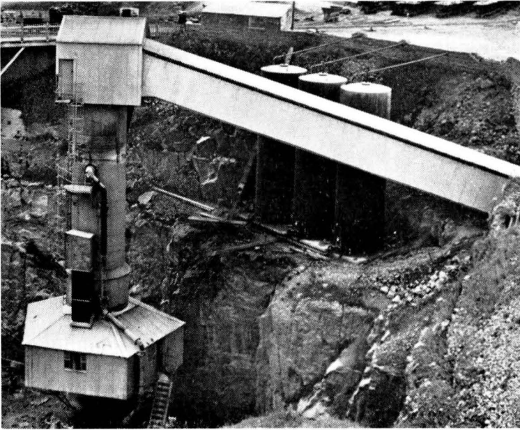
Fig. 8.—View of Kiln showing Raw Material Conveyor Gantry.
