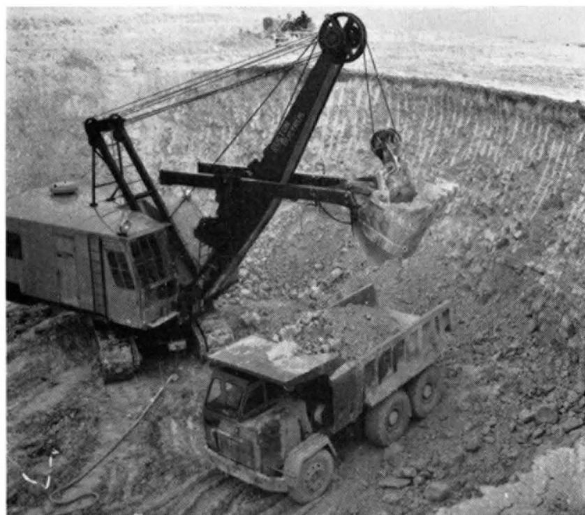
Fig. 3.—Loading in Chalk Quarry.
