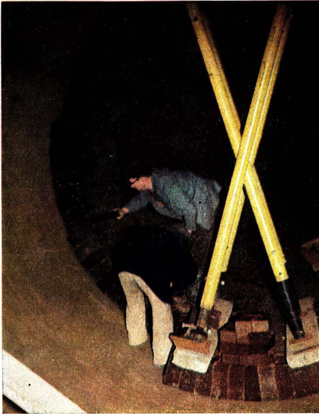
Kiln lining in progress with Magnesite/Chrome bricks
