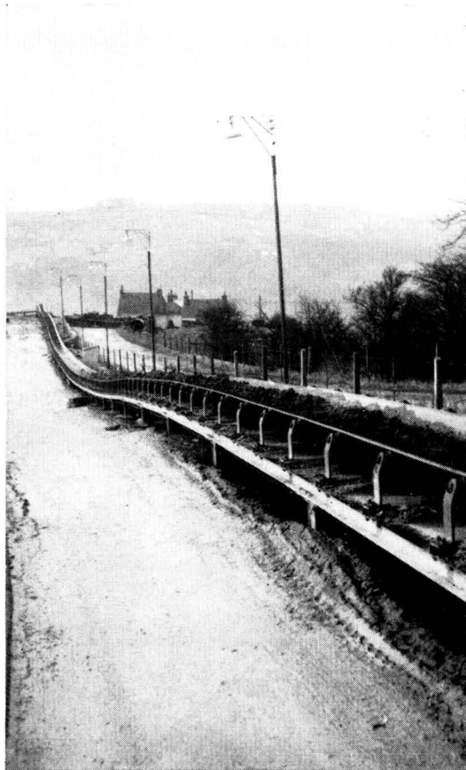
◀ Meco 2,000 ft. long Suspended Idler Belt Conveyor.
