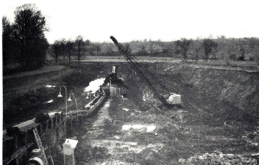
Fig. 5.—Drag-line and Conveyor in Clay Pit.
