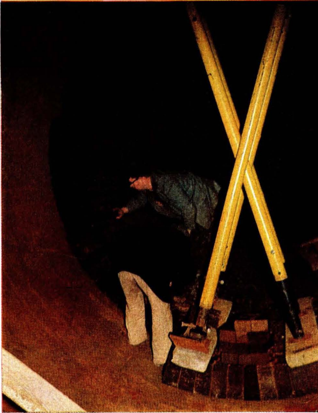
Kiln lining in progress with Magnesite/Chrome bricks
