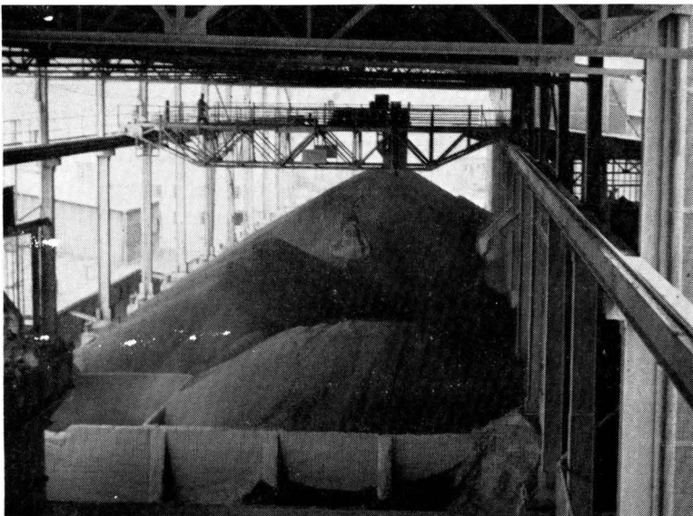
Fig. 6.—Cement Works, Jordan : Clinker Store.
