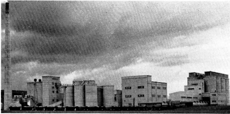
Fig. 22.—General View of Dunbar Cement Works.
