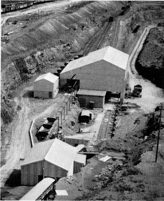
Fig. 4.—Quarry: Tipping Stations for Limestone and Shale, and Crusher House.
