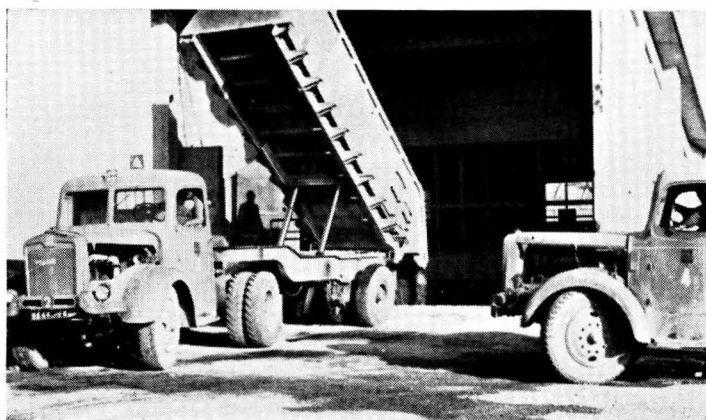
Fig. 5.—Discharging Raw Material at Bizerta Works.
