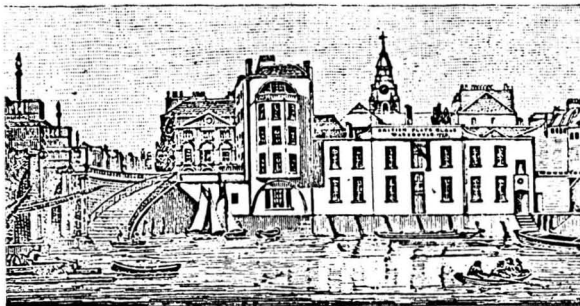
BRITISH PLATE GLASS WAREHOUSE, 1773, AT BLACKFRIARS.
