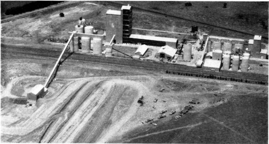
Fig. 1.—General View of Quarry and Works at Waurm Ponds.
