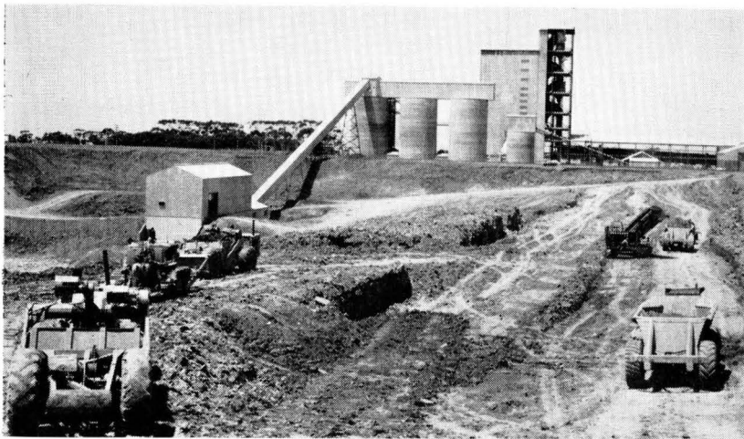
Fig. 2.—The Quarry: Stripping in Progress.
