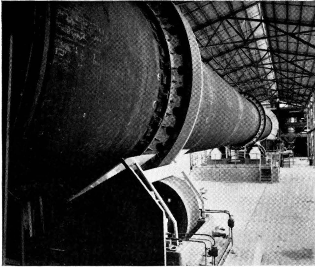
Fig. 6.—The Kiln House.
