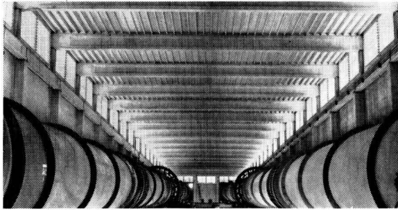
Fig. 14.—Kiln House with Prestressed Concrete Roof.
