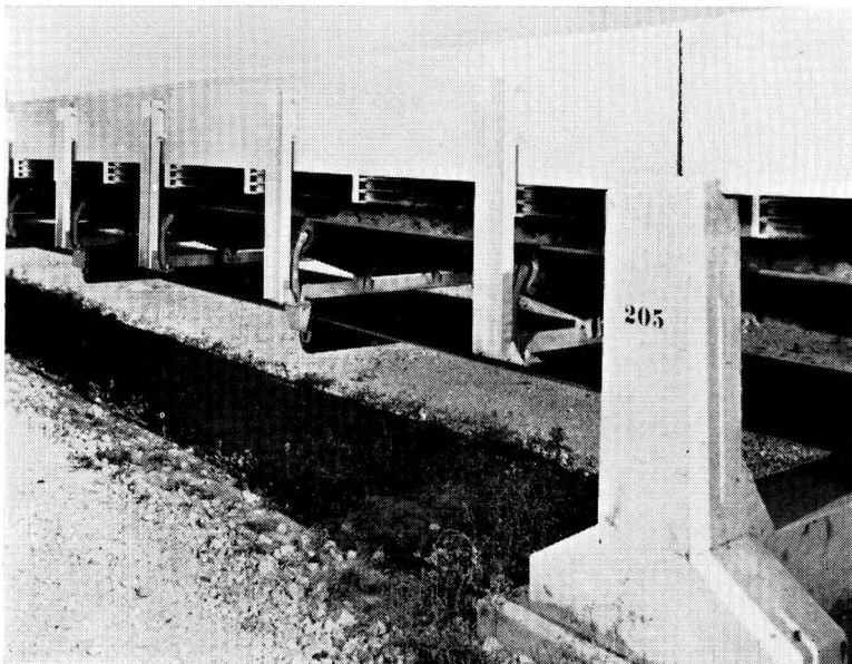
Fig. 21.—Concrete Structure for Conveyor at Ground Level.
