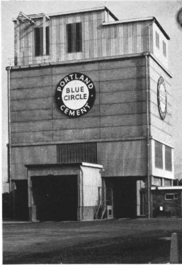
Fig. 6. Silo at Distribution Depot at Inverness.
