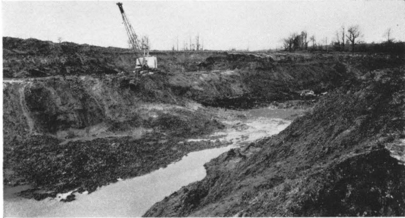
Fig. 3.—Excavating at Clay Pit.
