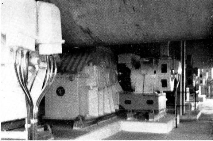
Fig. 14.—Kiln-drive Motor and Gear-box.
