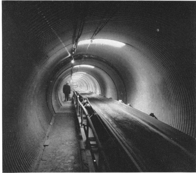
Fig. 8. Interior of Conveyor Tunnel from Quarry to Works.
