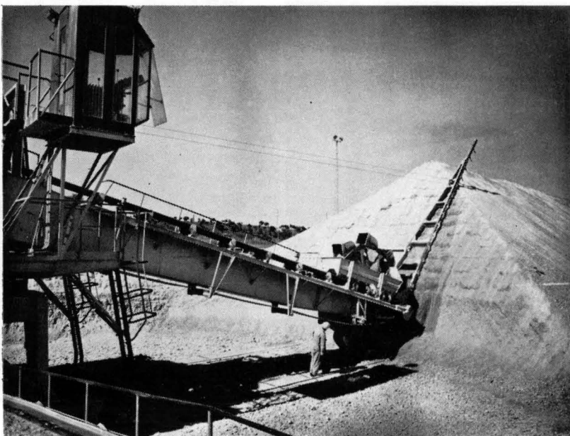
Fig. 7. (Below) Bucket-wheel Excavator for reclaiming Raw Meal.
