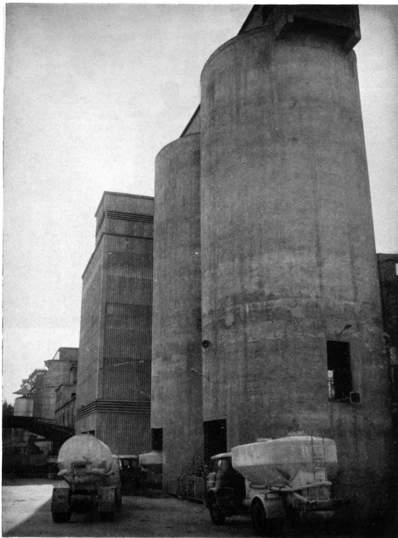
Fig. 12.—Cement Silos and Despatching Plant.
