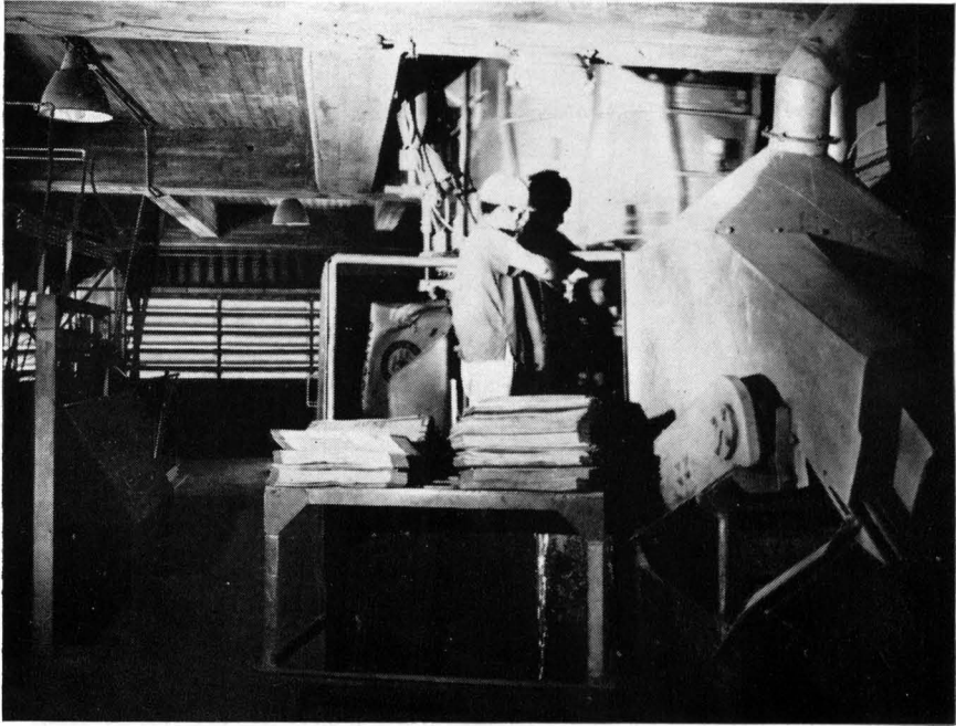
Fig. 13.—Eight-spout Rotary Packer.
