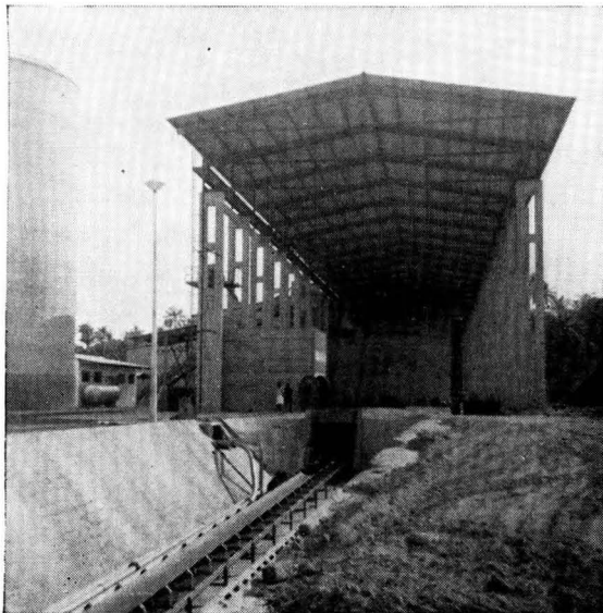
Fig. 7. — Materials Store (showing Clinker Conveyor to Wharf) at Calabar Works.
