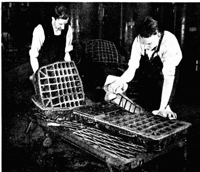
Manufacture of Sponge Rubber Automobile Seats : Opening the Moulds
