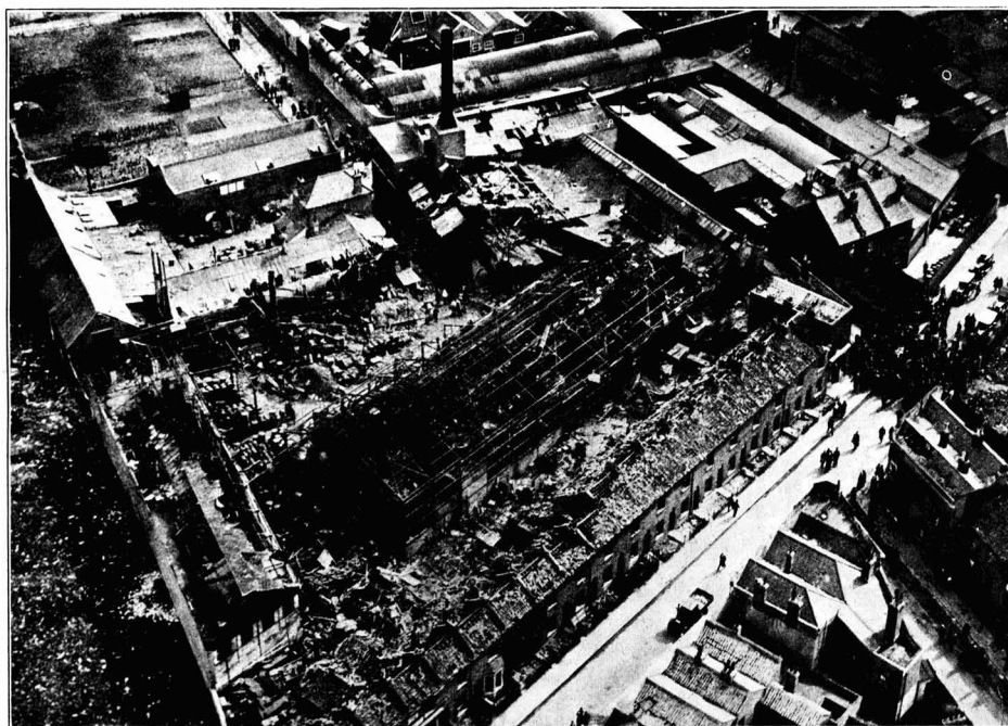
An aerial view of the Mitcham Chemical Works of W. J. Bush and Co., Ltd., after the explosion, showing the extent of the damage to surrounding property.
