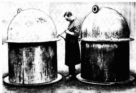
The same Pans successfully repaired by Scientific Welding, the centre flanges being cut away and new ones welded on.
