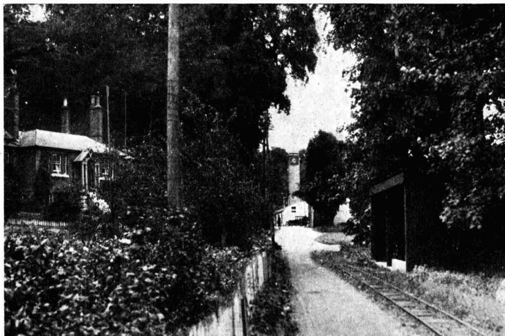
The Foreman's House at Oare Works is set against the side of a Wooded Hill. In the background is the Old Clock Tower.
