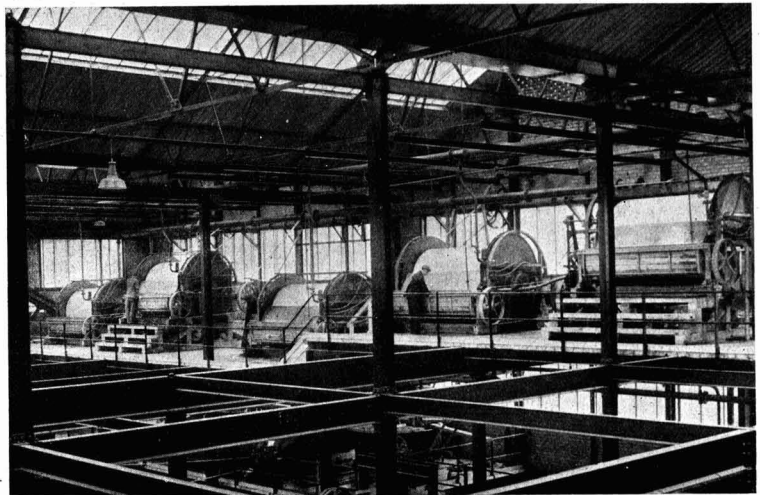
This Battery of Washing and Filtering Machines is an important feature of the new works.
