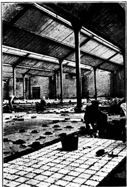
Above: KaBe acid and alkali resisting flooring in course of being laid. Right: KaBe products are used in the construction of this copper recovery plant.
