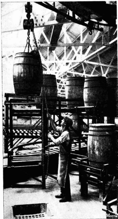
Above: Rapid transport for barrels is provided by this Morris Conveyor, whilst a Morris Runway assists in handling the barrels when discharging the contents through a chute in the floor.
