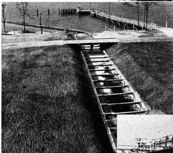
Below.—Effluent sea water passing from blowing-out Towers to river.
