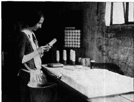
Making Soxhlet Thimbles from wet pulp. These thimbles are used for testing the purity of milk.
