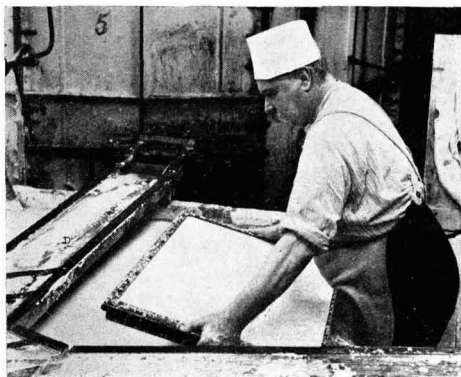
Vatman dipping the mould into the vat.
