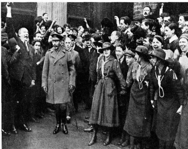
His Majesty the King visiting the works of George Kent, Ltd., November 1917.
