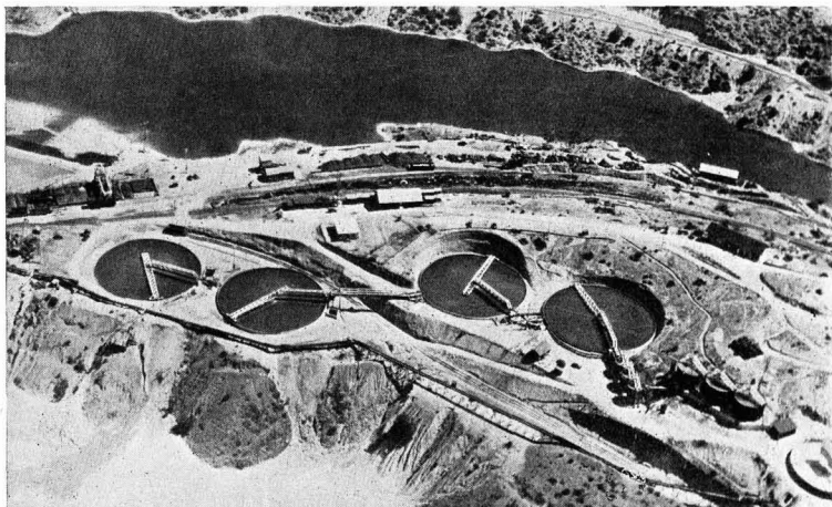
The Copper Leaching Plant of the Inspiration Copper Co., U.S.A., with Dorr thickeners and classifiers, pumps, mixers and agitators, all of acid resisting construction.
