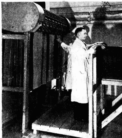
The sheets being placed in the dryer. All that remains is for them to be cut, inspected and packed
