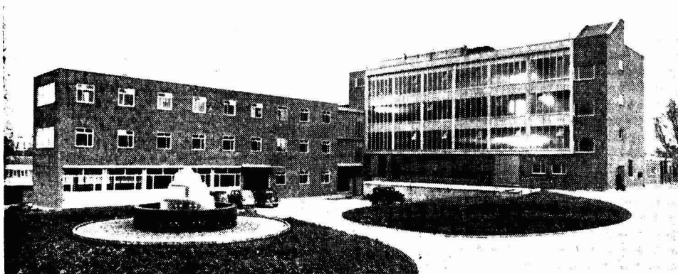
A view of part of the new factory showing the building housing the blower and refrigeration plant (right) and the office and laboratory block (left)
