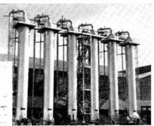
INDIA. Six carbon dioxide scrubber towers 75 feet hlgn wash a stream of gas under a pressure of about 300 lbs, per sq. inch.
