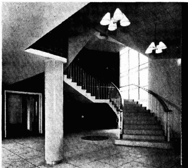
Fair-faced brickwork covers the white acoustic ceiling tiles and white plaster walls in the entrance hall. The cantilever stairway is finished with terrazzo treads, white baluster rails with polished mahogany handrails in natural colour and backed by plaster finish walls painted in dark blue
