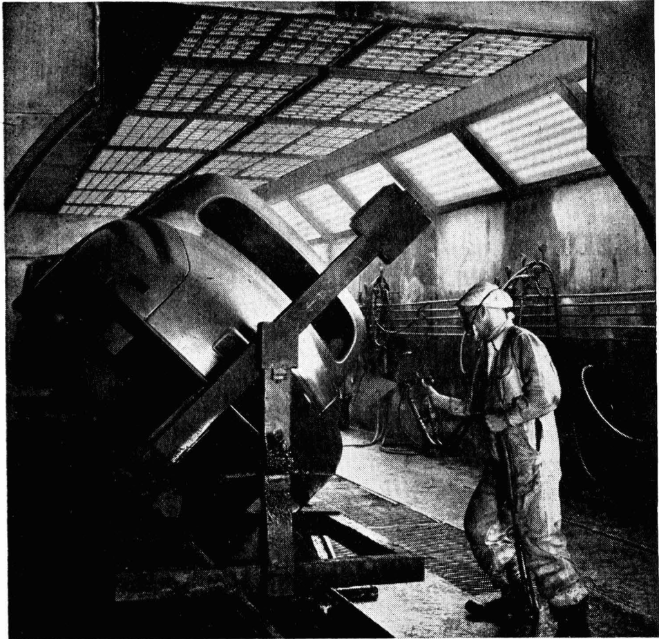
Rover Car Factory, Solihull. High intensity lighting in a body spray tunnel by fluorescent lamps in a glazed enclosure.
