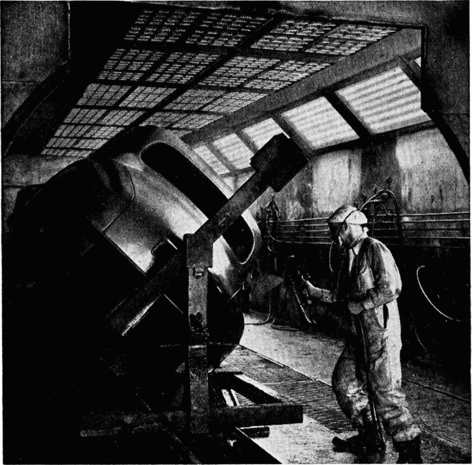
Rover Car Factory, Solihull. High intensity lighting in a body spray tunnel by fluorescent lamps in a glazed enclosure.
