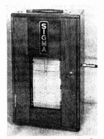
Sigma Mark V recorder for indicating and recording pressure or vacuum
