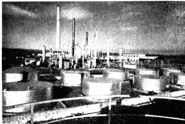
Storage tanks, topping plant No. 1, and cracking plant in the Augusta refinery
